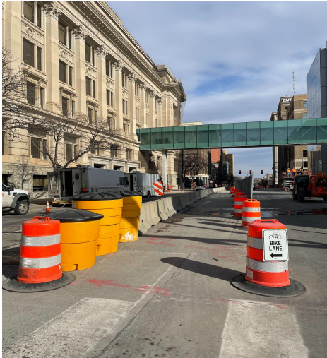
Image 8: Construction detour between 17th & 18th Streets
